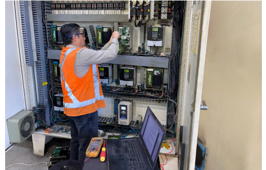
CCI Senior Control Field Engineer commissioning Yaskawa drives.
